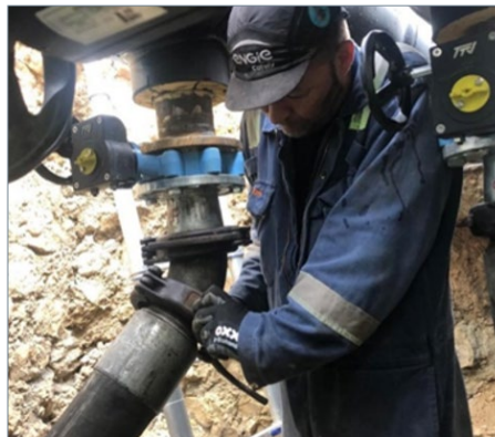
Fig. 17 – Installation of Flexible Hose on pre-installed DN100 Offtakes
