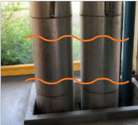
Fig. 9 – Sections for removal (feeder & return line)
