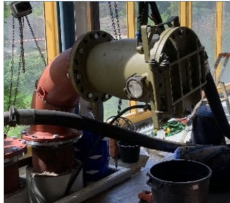
Fig. 15 – Completed Setup at Boiler Plant Including Hoses and Temporary Piping Connected to Quest Pump Unit
