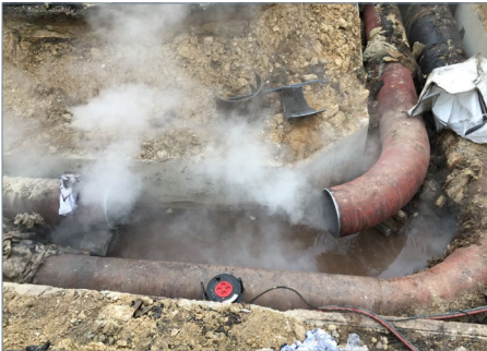
Fig. 6 - Section of pipework removed following leak
