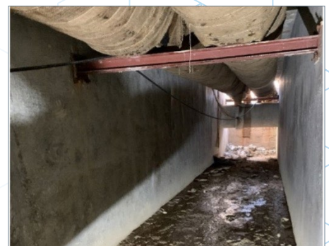
Fig. 5 – Feeder and return pipes supported within concrete channel
