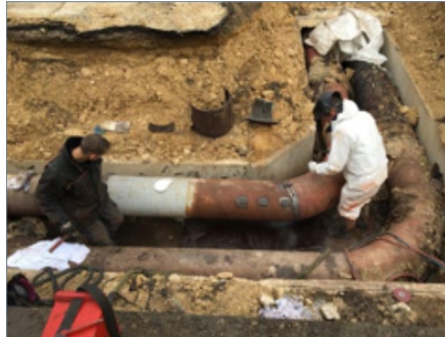
Fig. 7 – Finalization of repair using replacement pipe
