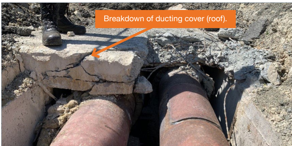
Fig. 8 – Cross section of broken-down ducting cover enabling water ingress
