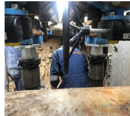
Valved Offtakes Installed to Feeder & Return Line 1km Downstream From Boiler Room
