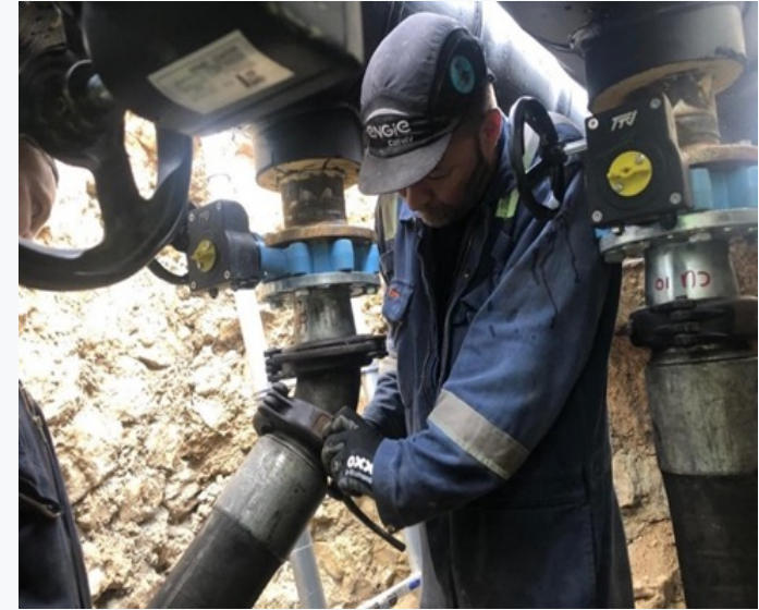
Looping of Feeder & Return Line
