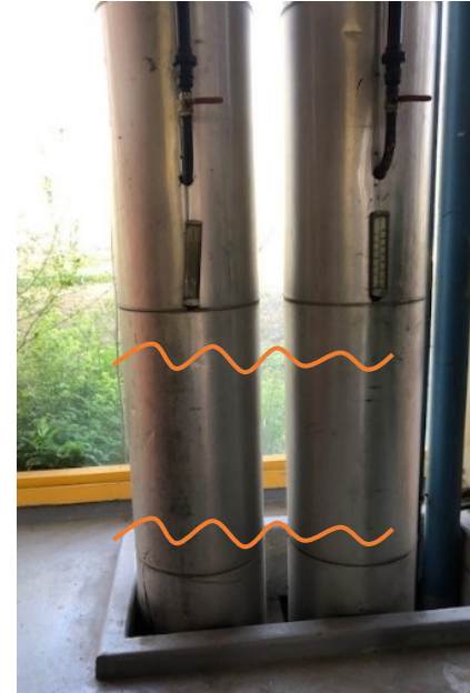
Section of Piping To Be Removed From Feeder & Return Line in Boiler Room
